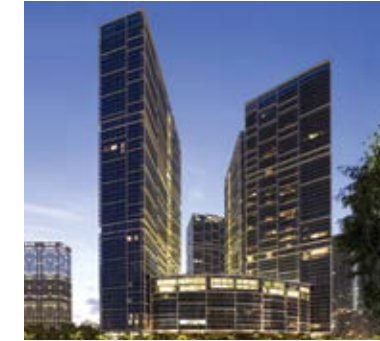
Icon Brickell Condominium + Viceroy Resort Miami, Florida
